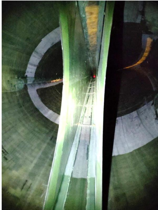
*Figure 1: Inside of 45m blade of an ESM-owned turbine with two webs.*
