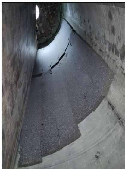
*Figure 6: 12m<sup>2</sup> noise-absorbent mats of 5cm thickness at the blade root of 57m long blade.*
