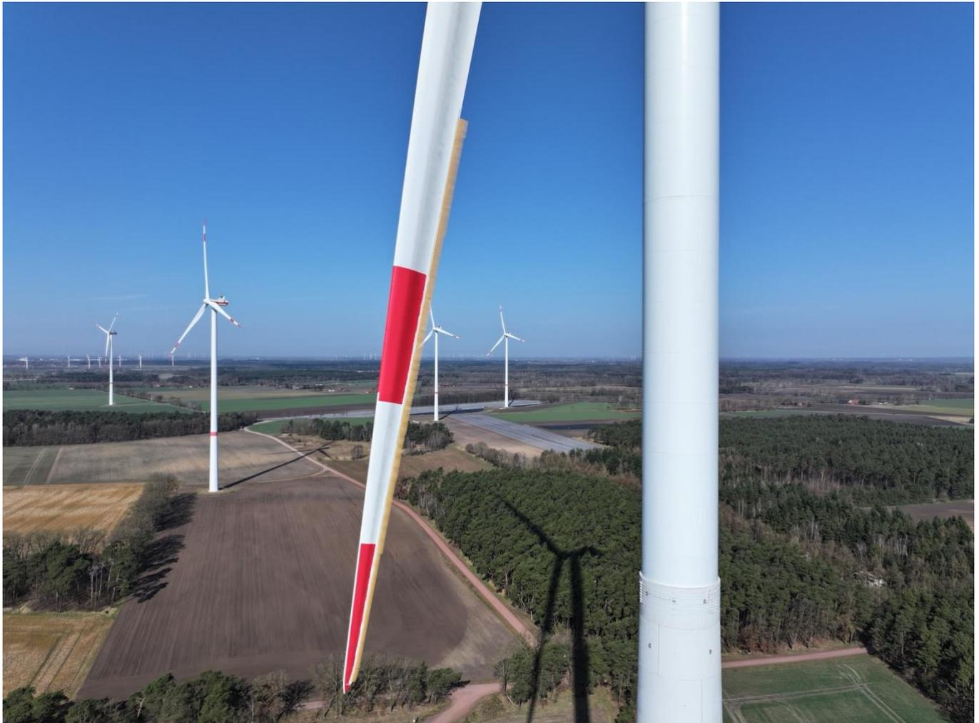
*Figure 1. An aerial shot of the FeatherEdge® technology installed on the ENERCON E160 EP5 E3 at Hämelhausen, Germany (Credit: Schierloh Engineering GmbH).*
